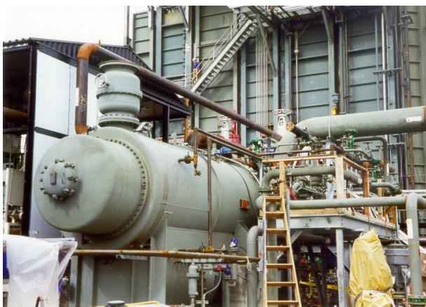
Figure 1. Turbine exhaust steam surface condenser (straight tubed vacuum condenser).
