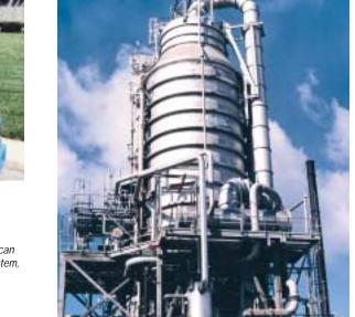
Vacuum precondenser on a visbreaker at a South American lube oil refinery. Vacuum system supplied as unitized system,
