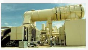
A large stainless steel condenser for a geothermal power plant on the U.S., West Coast
