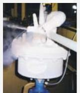
A cryogenically cooled vent condenser at a chemical storage facility that reclaims 98 percent of VOC vapors as condensate.
