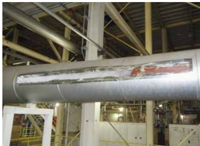
Figure 1. Insulation removed from the first stage ejector, showing frost formation. Source: Graham Corporation
