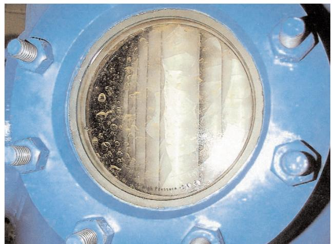
**Figure 3c. End of cycle (when there is substantial ice buildup)**
