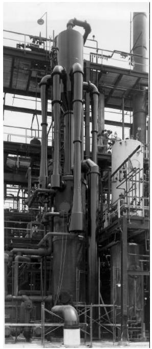
Figure 5. Steam Vacuum Refrigeration Unit
