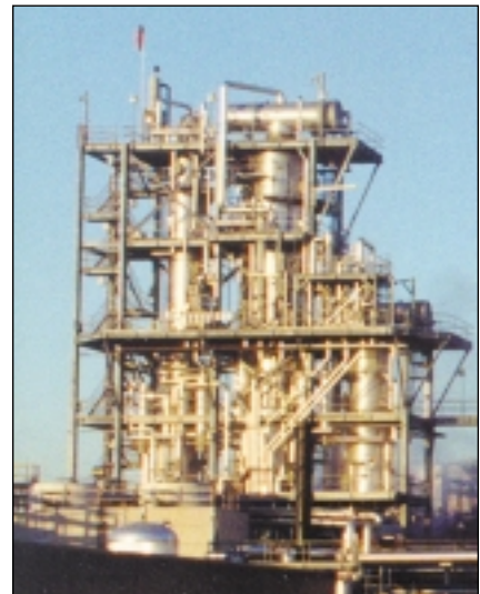
Fatty alcohol distillation column with the vacuum condenser attached directly to the distillation column. No piping or pressure drop between the two components.
