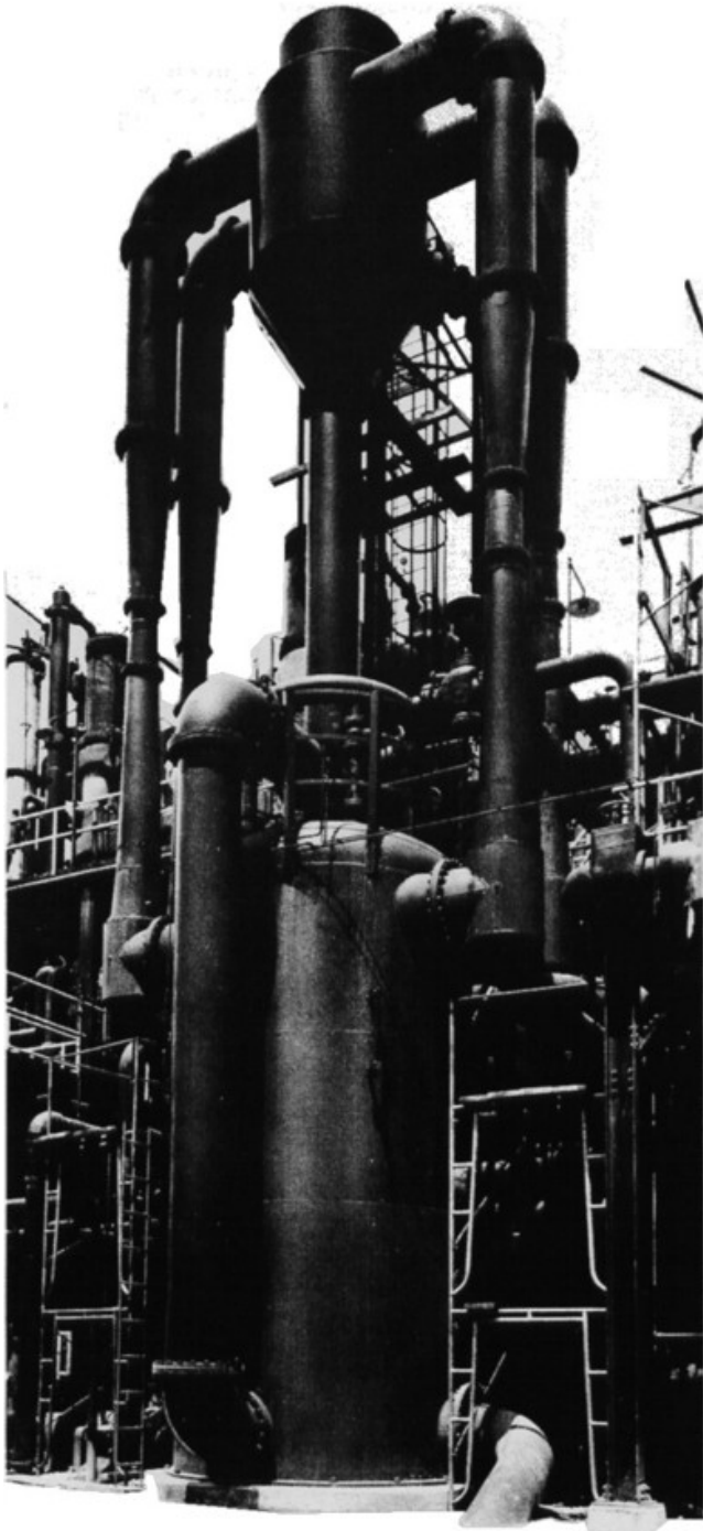
One of the largest. Modern chilled water system in large chemical plant.
